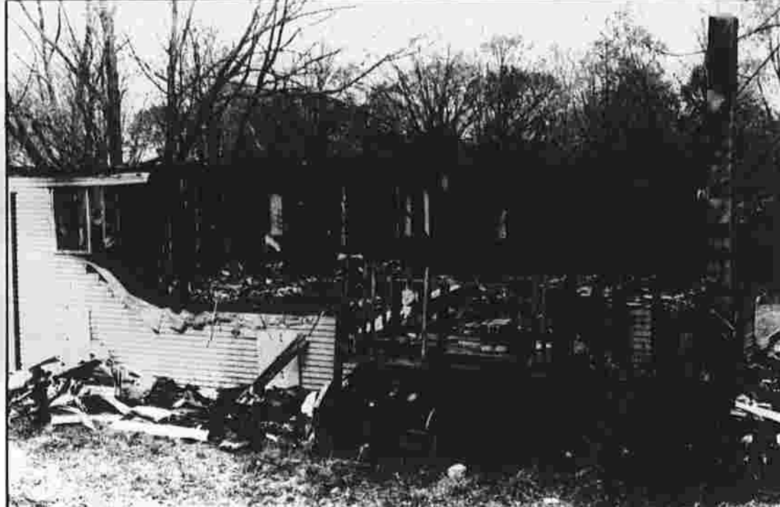
SUSPICIOUS BLAZE — The foundation of a home at 10 Skinner Hill Road in Andover is all that is standing today after a suspicious fire Saturday. The Bureau of the State Fire Marshal is investigating the blaze. Story on page 1.
